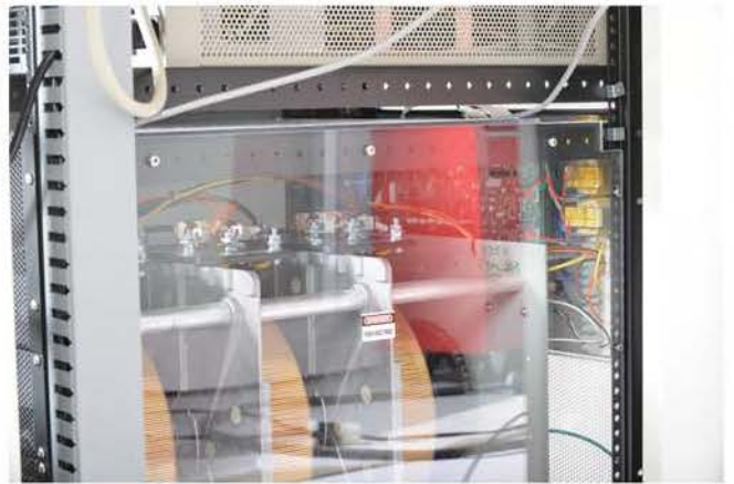
3 Phase 400 Hz Motor Driven Transformer
