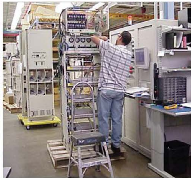
Connecting a Power Cabinet for Test
